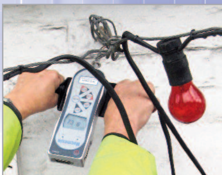
Pull test on anchorage points
